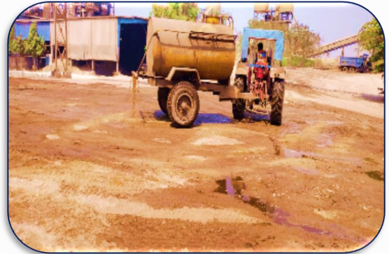
Dust Suppression by Dustex
