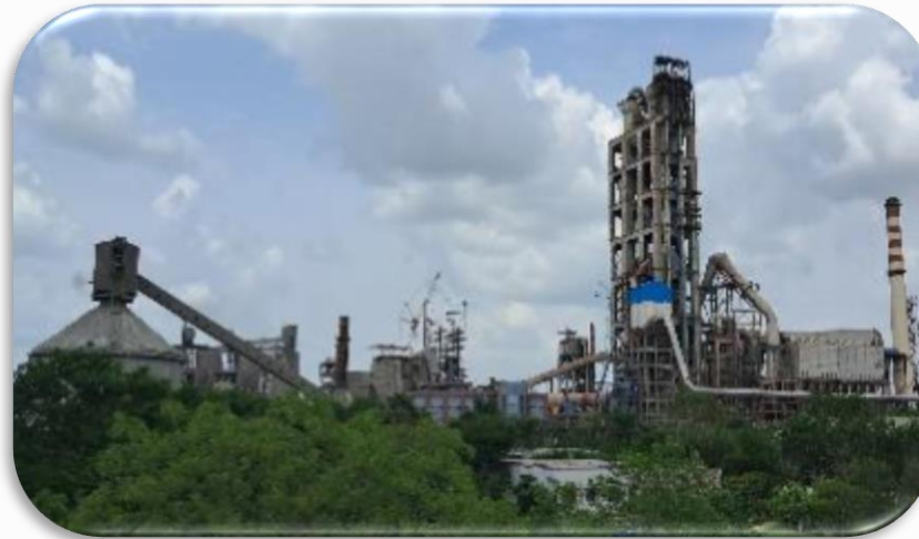
Dense plantation in plant area
